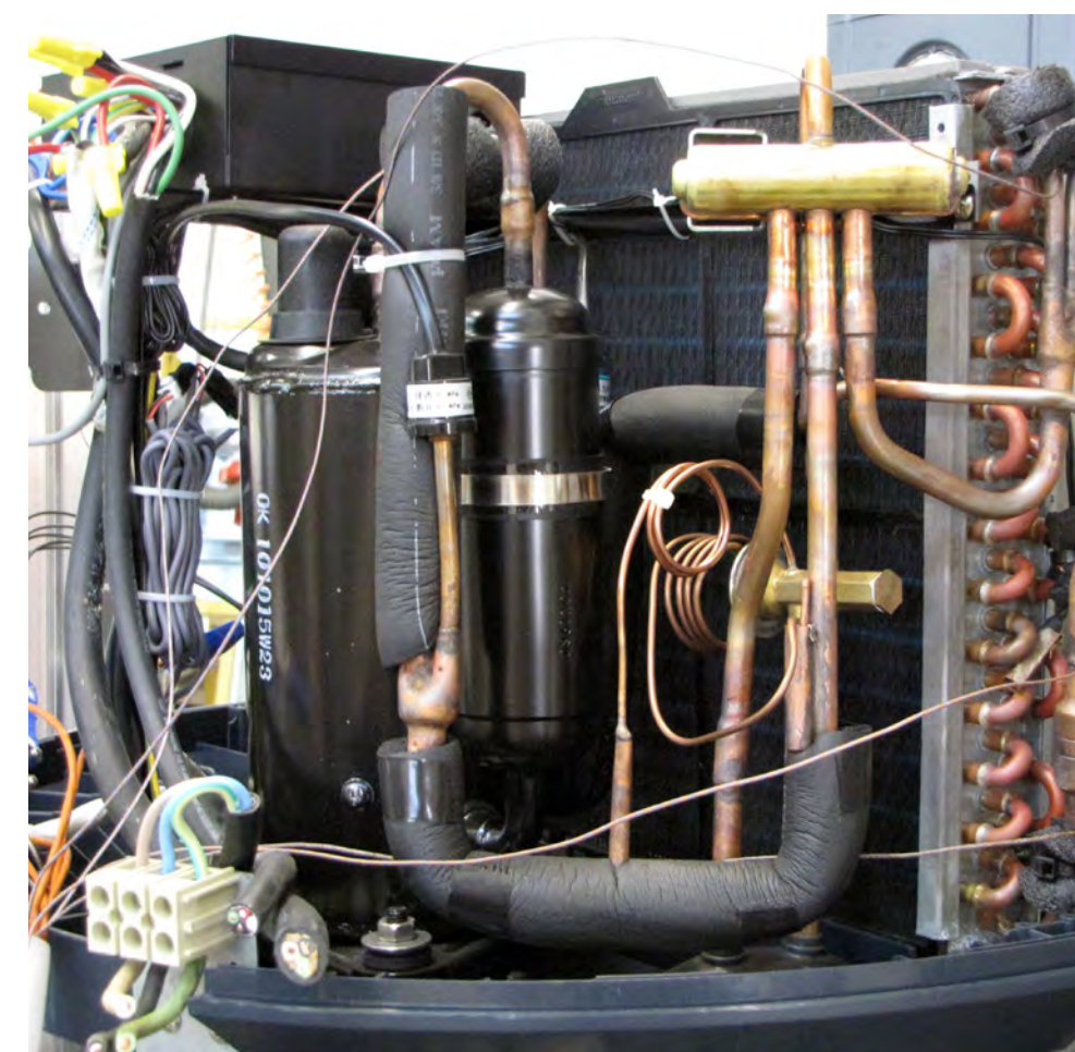
Interior components of a packaged heat pump.
